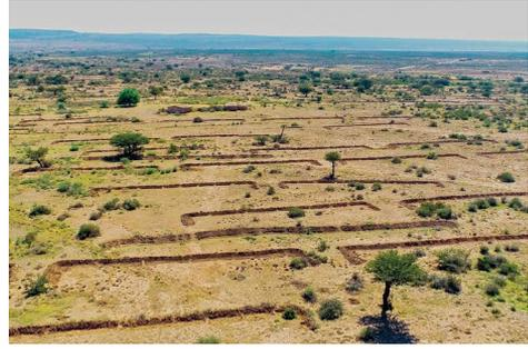
*Constructed soil bunds to reduce water runoff and soil erosions near Karin village, Sanaag region*
